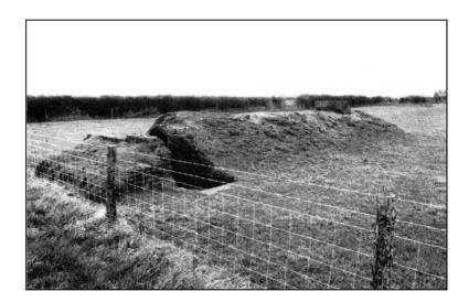
Fig 19 Photograph of a 'Stanton' semisunken shelter
