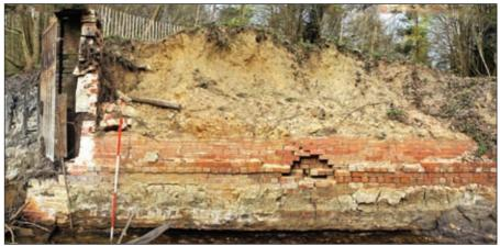
Photograph of west face of dam, showing the brick culvert.
